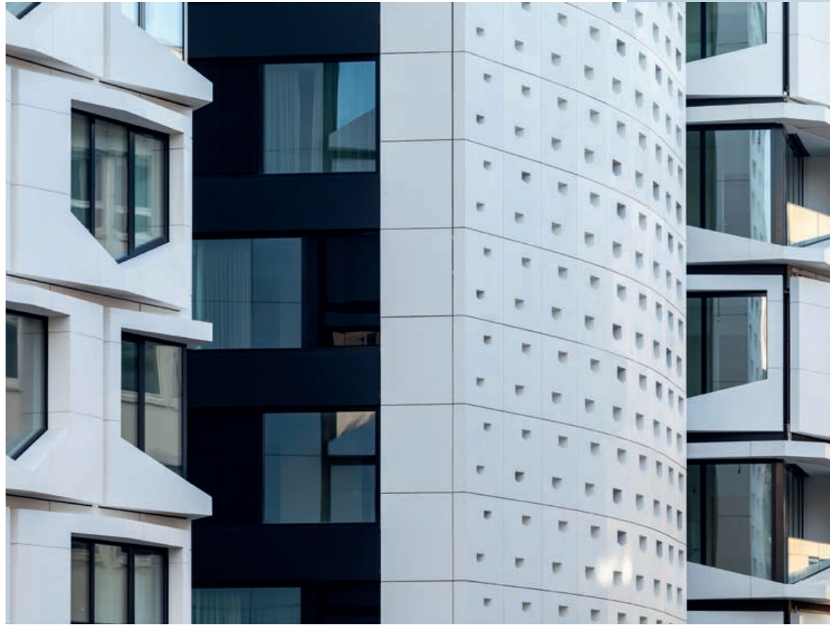
FLARE OF FRANKFURT, Frankfurt, (Germany)
