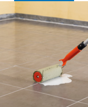
Application of Mapecoat I 600 W on tiles prepared accordingly
