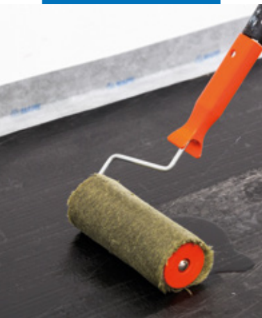
Application of Aquaflex Roof Premium on an old bituminous membrane
