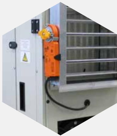
DAMPER WITH ACTUATOR AND ACCESS DOOR FOR FILTERS WITHDRAWAL
