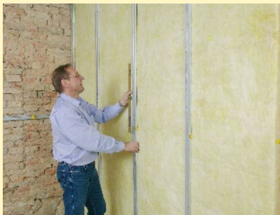
. Colocar la Lana Mineral ISOVER: CO 0 2.
