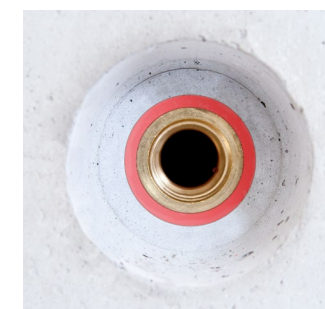
Illustration 3 Finished sprinkler connection in the concrete ceiling
