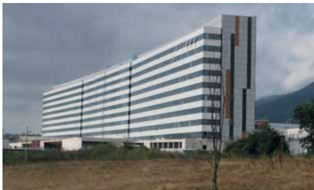
Hospital Central, Asturias
